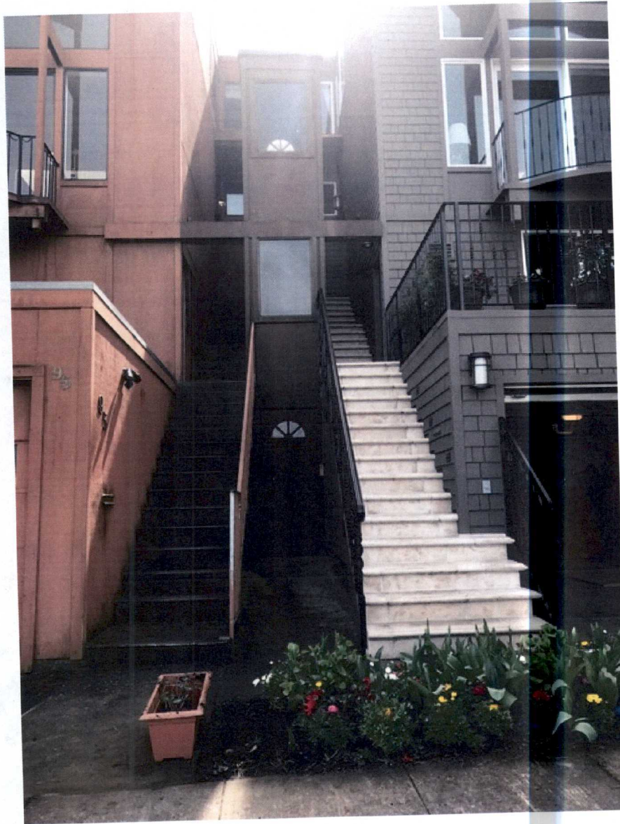
Elevator structure between 95 Saint Germain and 99 Saint Germain
