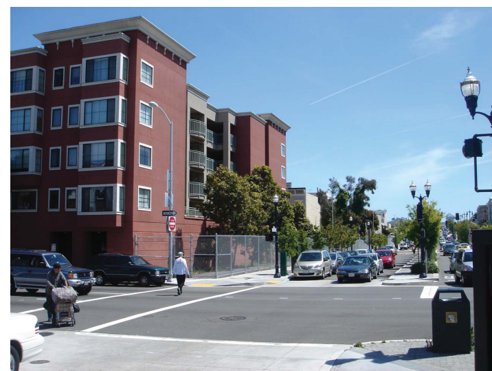
SITE M - OCTAVIA BLVD + FELL STREET - LOOKING SOUTH
