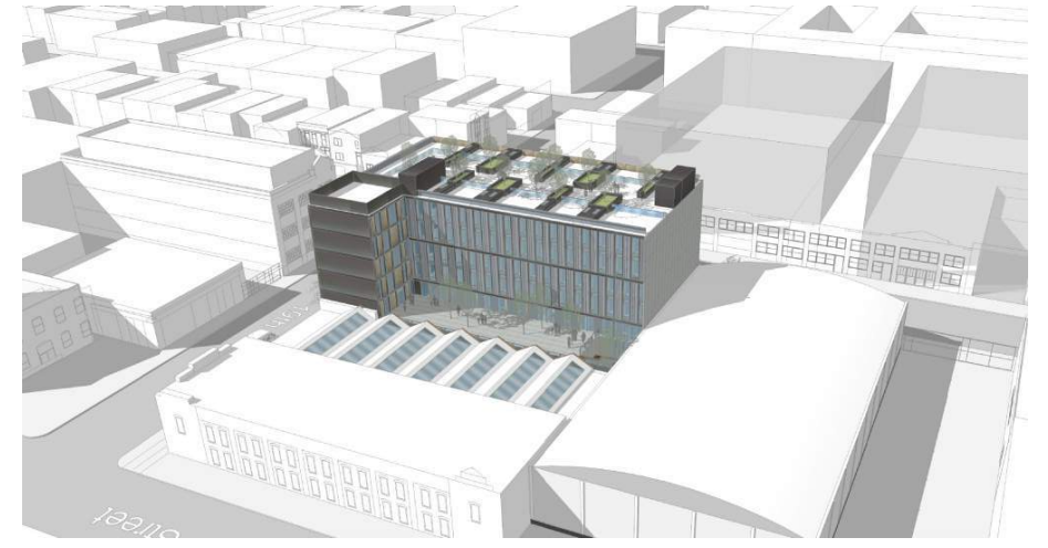
VIEW AT REAR OF BUILDING
