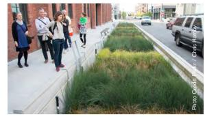
Sidewalk with Stormwater Planter
