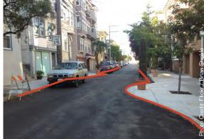
FIGURE 4.6.2: Example of Bulb-outs and Chicanes
