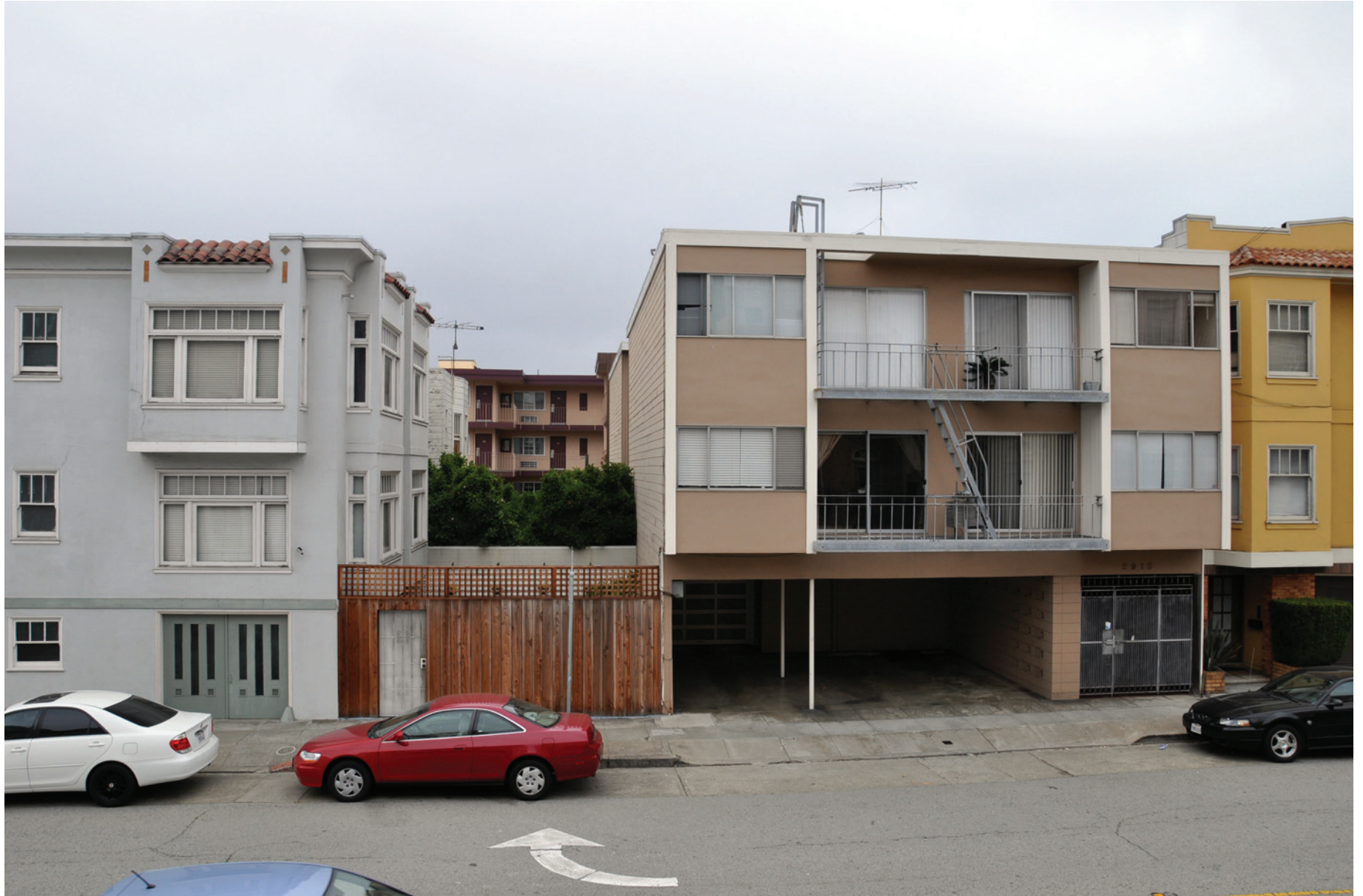
04 - FRANKLIN STREET FRONTAGE LOOKING WEST
