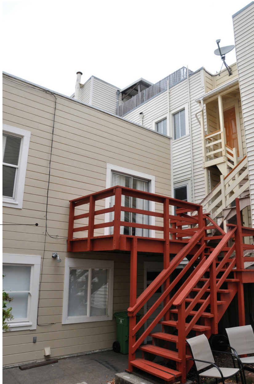
05 - REAR YARD LOOKING NORTH/WEST
