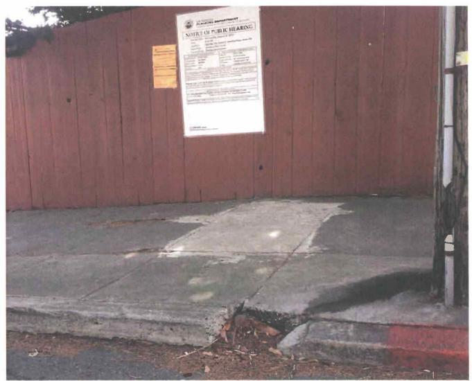
View showing sidewalk with small chunk of the curb missing probably having nothing to do with the trees, perhaps damage from the telephone pole. Usually old sidewalks are removed when a multi million dollar new home is built. This is an old sidewalk and complete speculation that the tree caused any damage. Conflicts between trees and infrastructure are common and removing a mature tree because of minor sidewalk damage is unacceptable.
