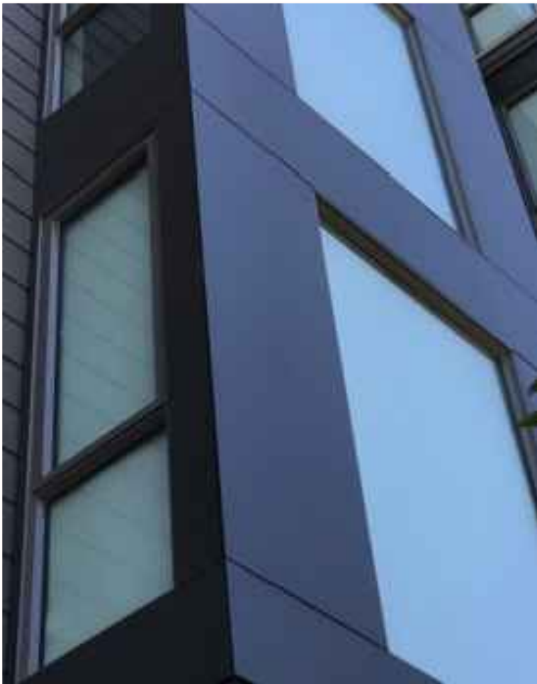
DARK GRAY METAL PANELING WITHIN STOREFRONT WINDOW SYSTEM AND SURROUNDING ENTER TO RESIDENTIAL LOBBY
