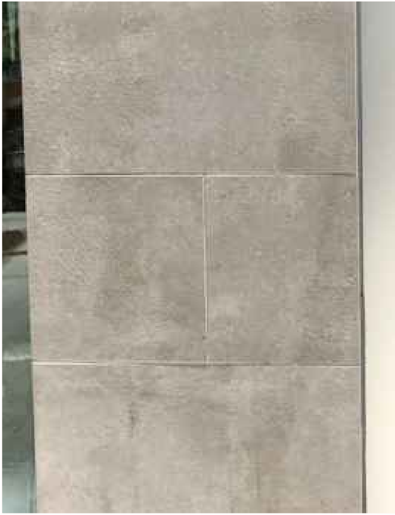
CEMENT GRAY TILE AROUND COLUMNS AND BELT COURSE ON RETAIL FRONTAGE
