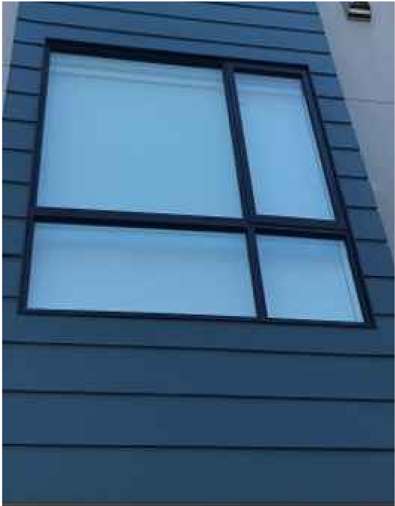
LAP SIDING ON ALL BAYS EXCEPT CORNER BAY
