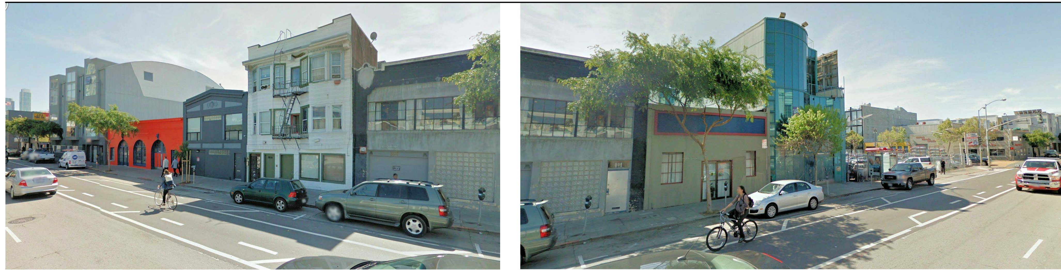
2 OBLIQUE VIEW OF BUILDINGS OPPOSITE THE FRONT OF 980 FOLSOM (VIEW FROM FOLSOM STREET)
