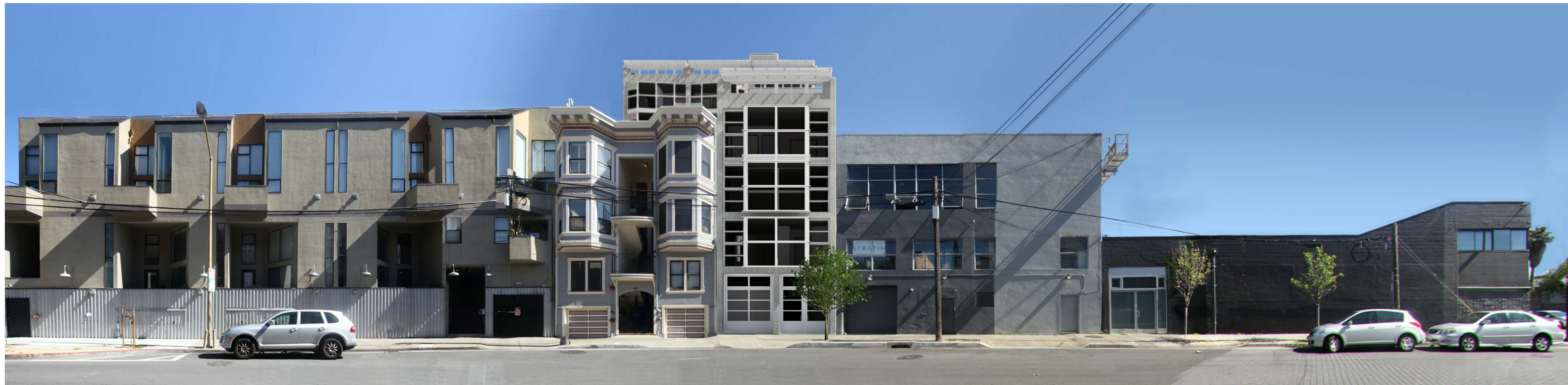
① PANORAMIC VIEW OF REAR OF 980 FOLSOM - NEW (VIEW FROM CLEMENTINA STREET)
