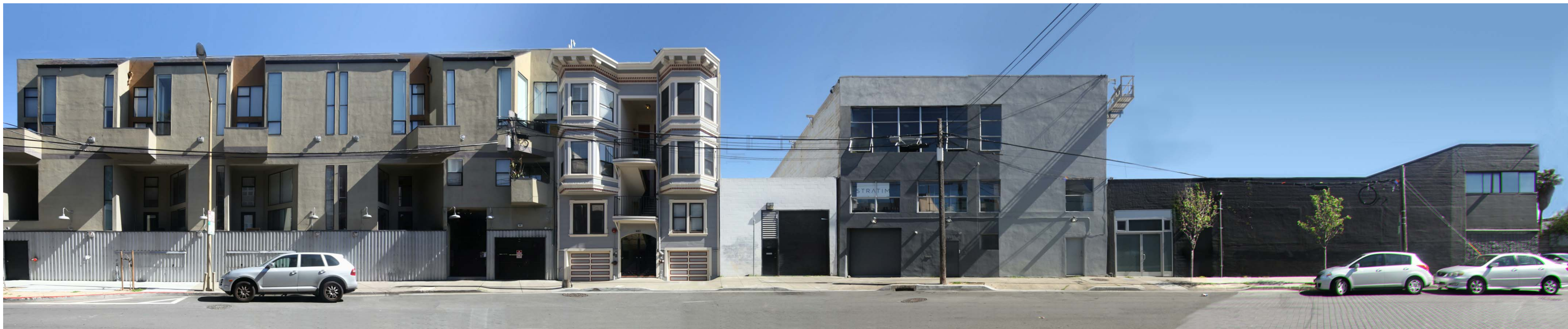
② PANORAMIC VIEW OF REAR OF 980 FOLSOM - EXISTING (VIEW FROM CLEMENTINA STREET)
