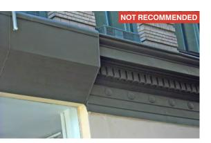
Removing, obsuring, or damaging historic features through installation of new features is discouraged, such as this historic beltcoursepartially concealed with an aluminum panel.
