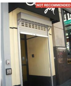
LEFT: When an external security grate is installed, its operational mechanism should be hidden from view. When fully retracted, the security grate should be concealed within the facade or behind the cladding.
