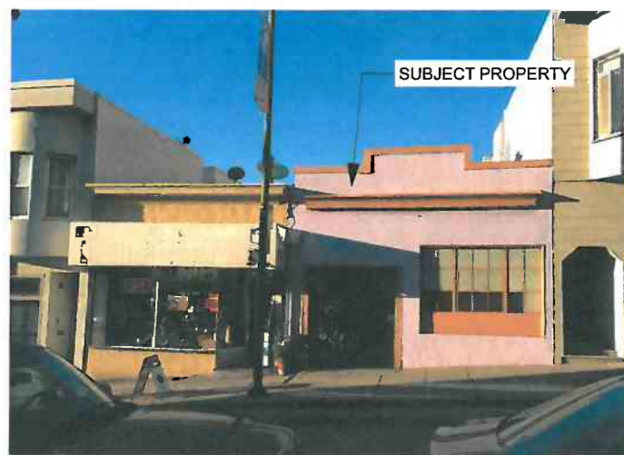
VIEW LOOKING AT FACADE OF SUBJECT PROPERTY
