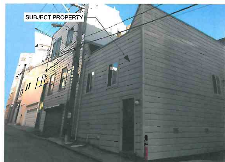
VIEW LOOKING EAST ON LYNCH ALLEY
