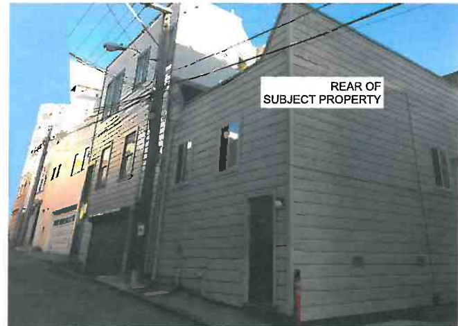
VIEW LOOKING EAST ON LYNCH ALLEY
