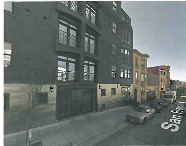
BUILDINGS ON THE FACING SIDE OF THE STREET
