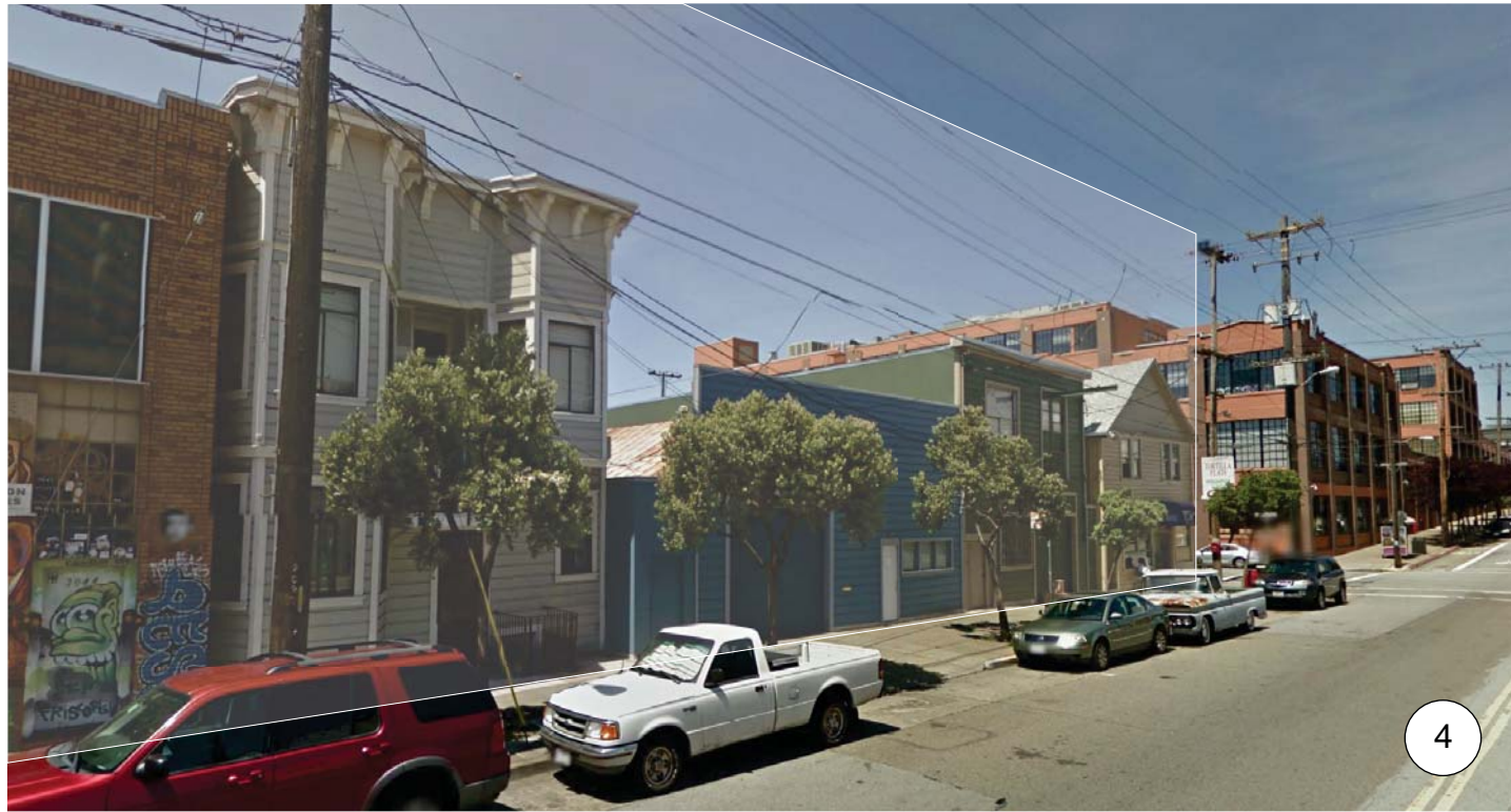
BRYANT STREET: VIEW NORTH TOWARDS 18TH STREET
