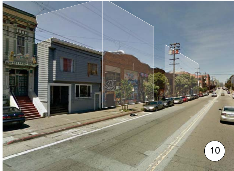
BRYANT STREET: VIEW NORTH TOWARDS 18TH STREET
