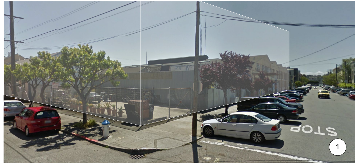
18TH STREET: VIEW SOUTH TOWARDS FLORIDA STREET
