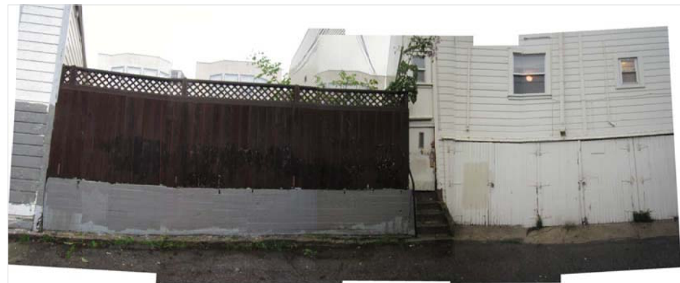
EAST SIDE OF QUANE ALLEY ACROSS FROM COTTAGE SITE
