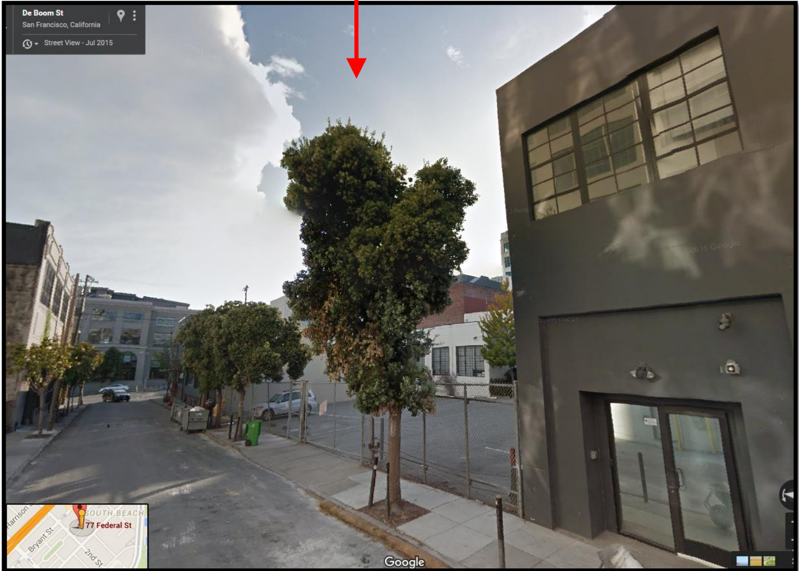
77-85 Federal Street, View along De Boom Street
