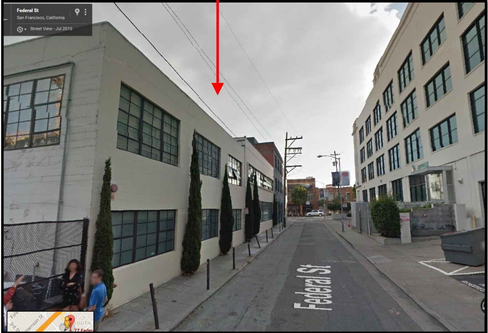
77-85 Federal Street, Existing Buildings along Federal St
