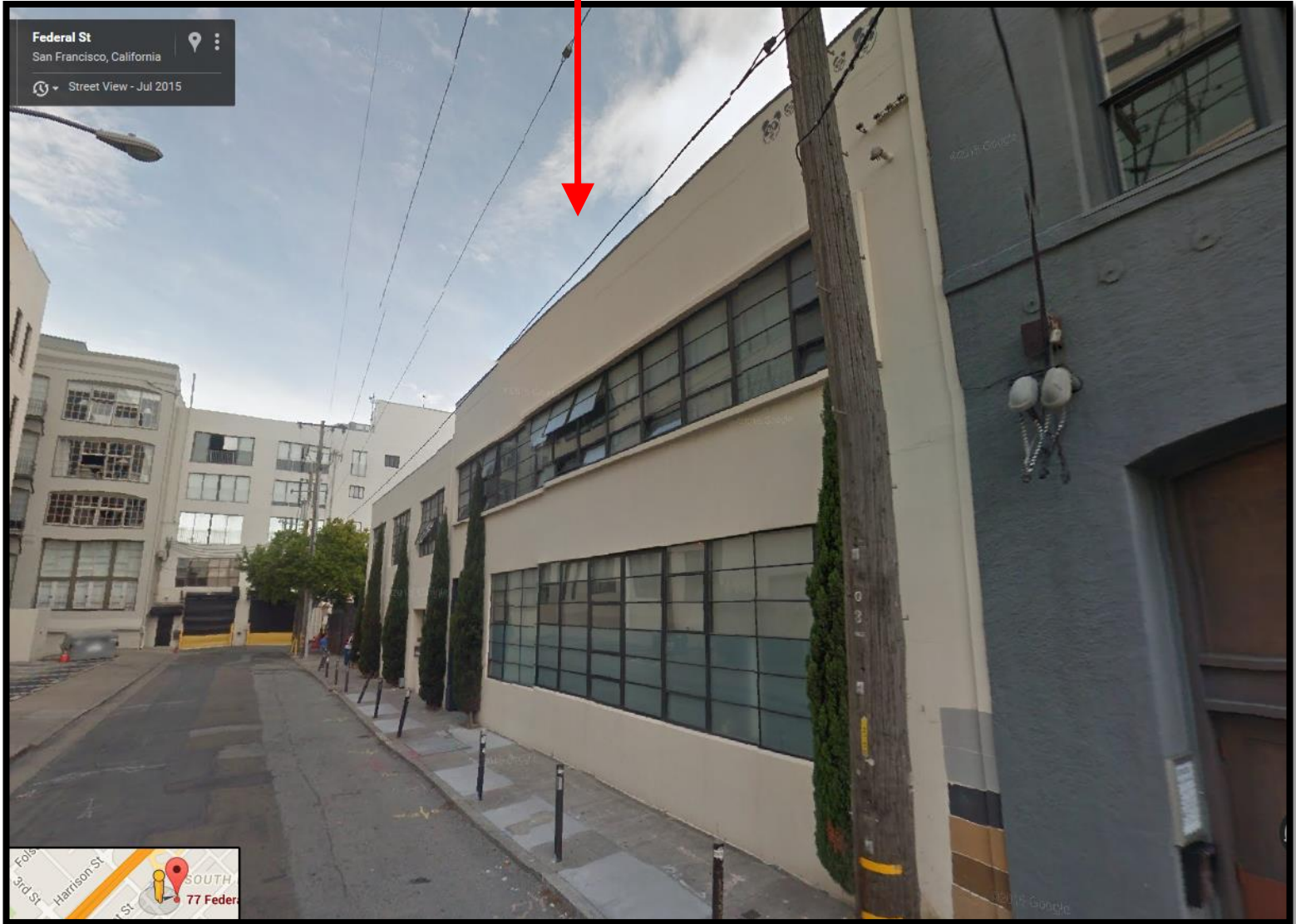
77-85 Federal Street, Existing Buildings along Federal St
