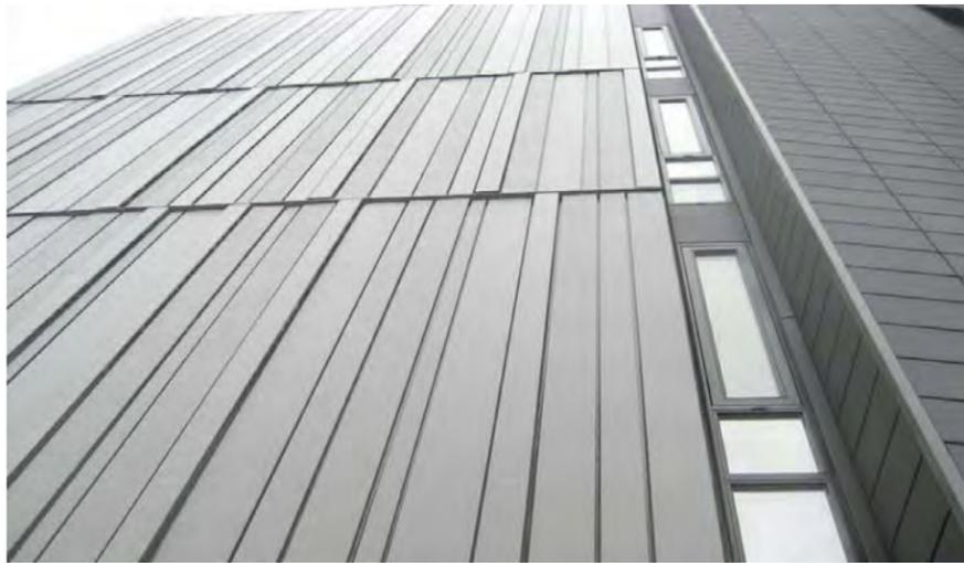
1) FIBER CEMENT BOARD (battens alternate in depth & width, painted light white)
