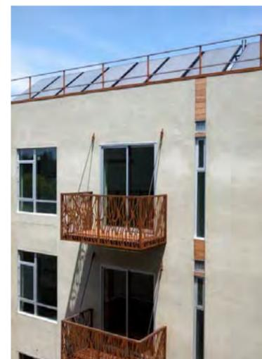
10) BALCONIES WITH CUSTOM CUT PATTERN OUT OF ANODIZED ALUMINUM (NOT CORTEN AS SHOWN)
