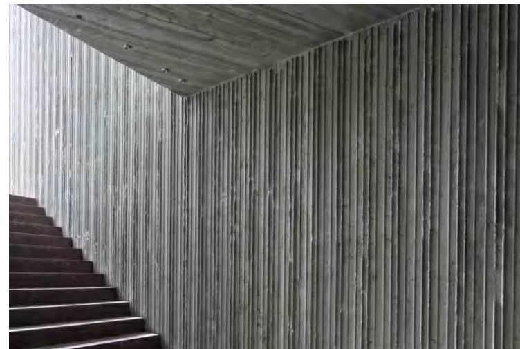
CORRUGATED CAST CONCRETE BASE ALONG 17TH ST.
