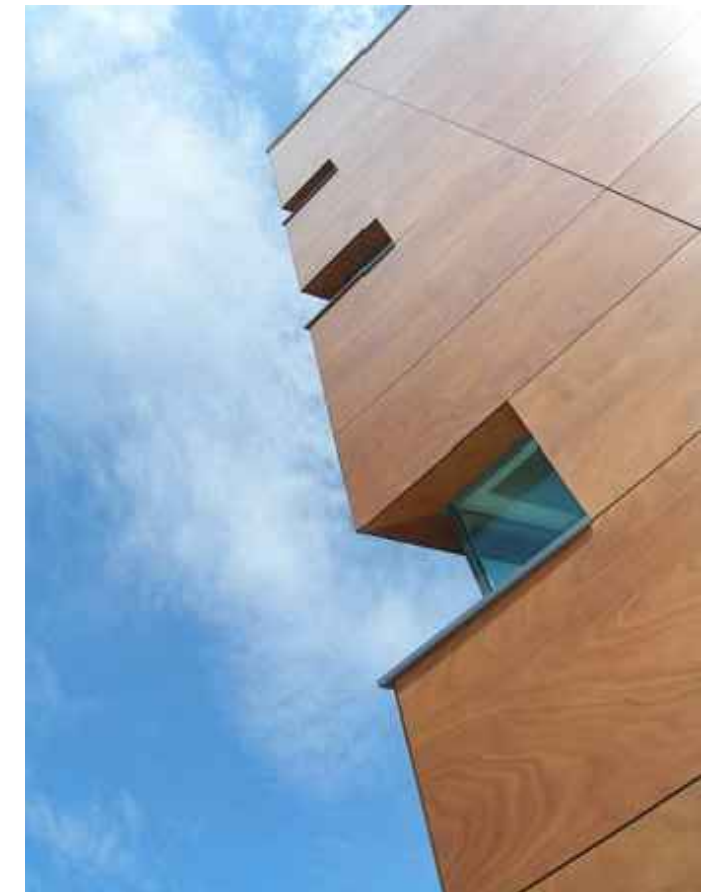
FIBER CEMENT PANEL ACCENTS AT BAYS
