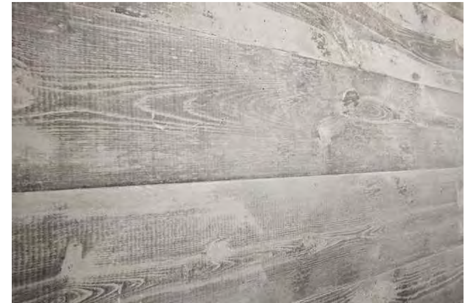
BOARD FORMED CONCRETE AT FIRST TWO LEVELS ALONG 17TH STREET
