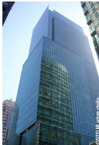
Fig. 1.5.2d Generation Four. 555 Mission St., 1988; Heller Manus; Height: 447 ft. Floorplate: 16,000 gross sq. ft.
