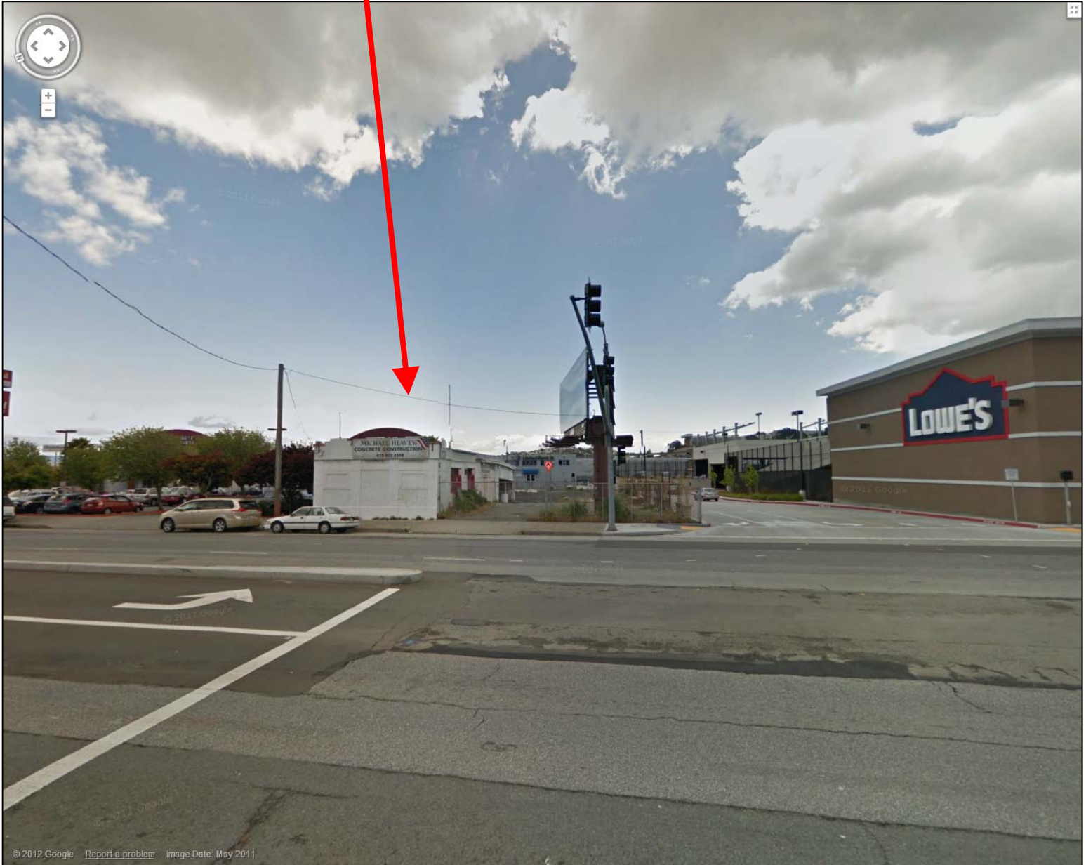
367 Bayshore Boulevard, View along Bayshore Boulevard
