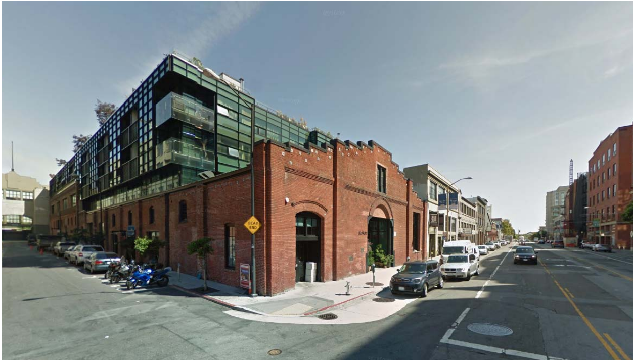
FIGURE 2.7 166–178 Townsend St (2016, After Construction)
