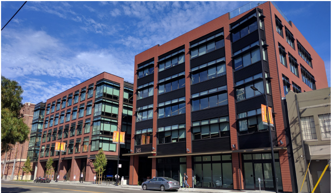
FIGURE 2.4 333 and 345 Brannan Street (2016, After Construction)
