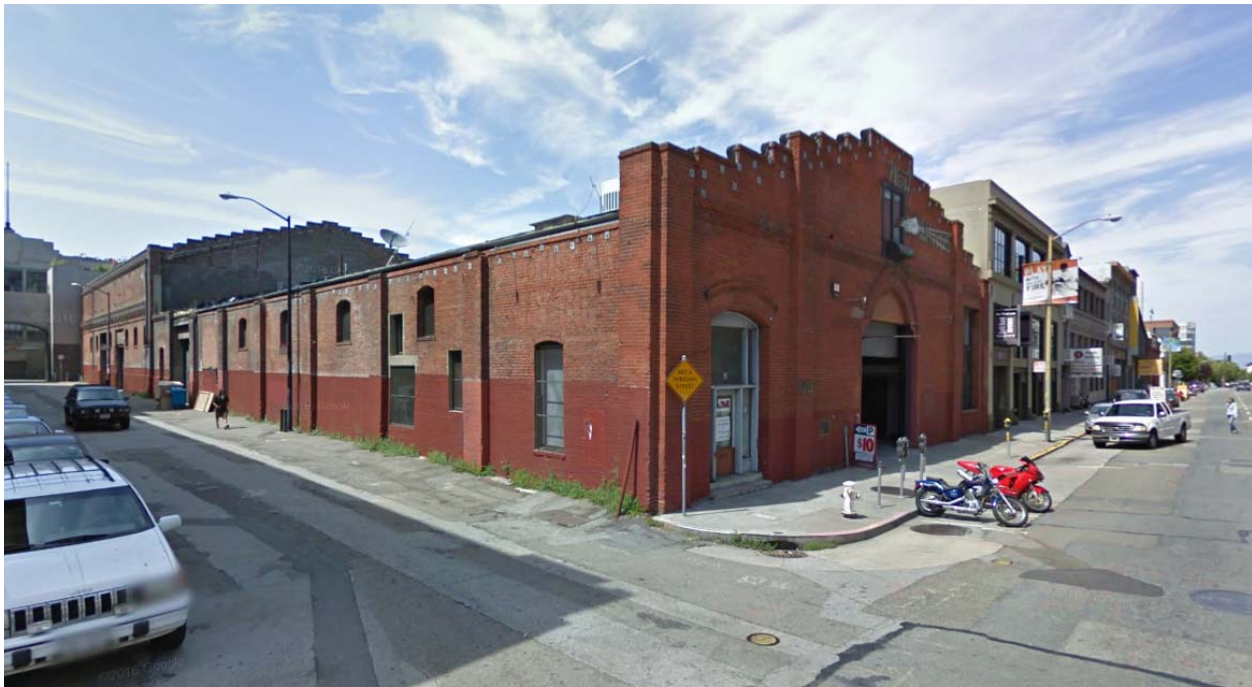
FIGURE 2.8 166–178 Townsend St (2009, Before Construction)
