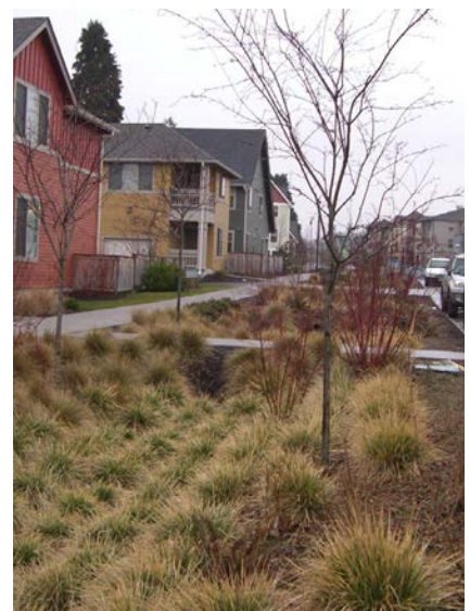
Biofiltration Swale
