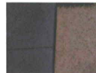
TEXTURED AND COLORED CONCRETE
