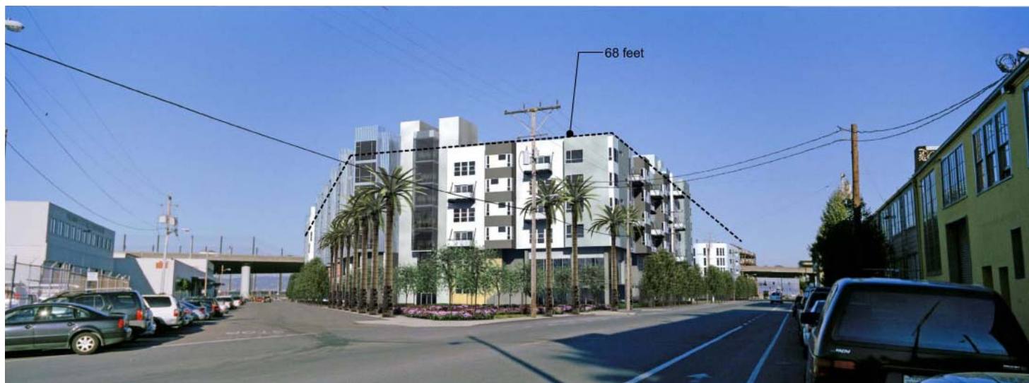
Figure C&R 3 – View B : Looking East from Hubbell and 16 th Streets Source: David Baker + Partners
